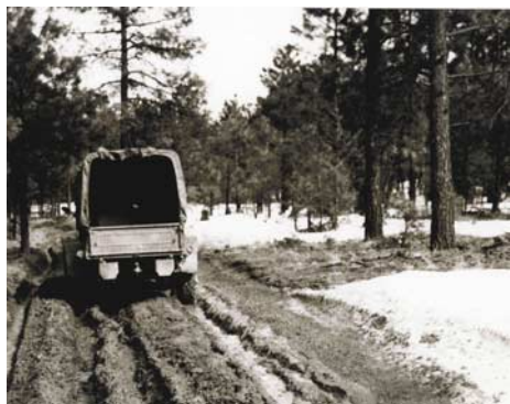
Typical muddy road in Los Alamos, NM
